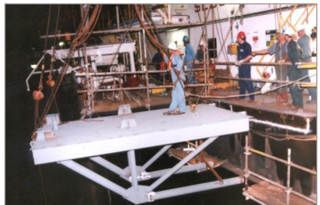
Lifting the new deck section into place
