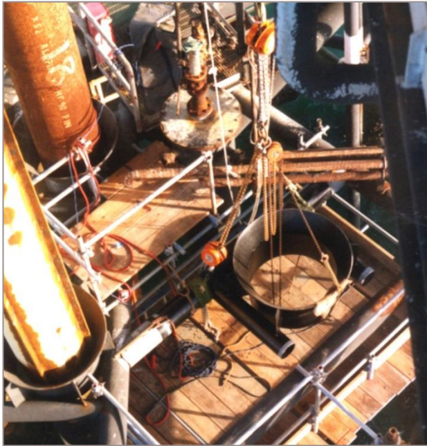
Installation of the conductor guide near sea level
