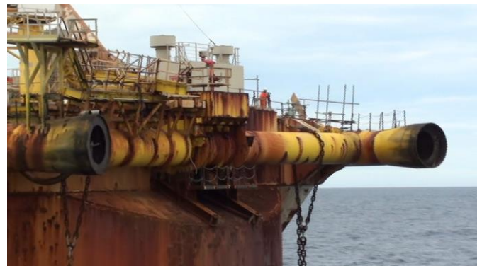
FPSO Yoke remnant
