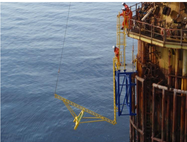
SALM ladders and platforms
