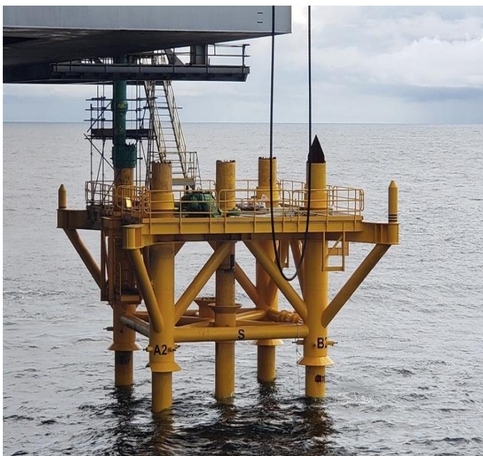
Conductor Supported Platform – Drill Deck Module.
