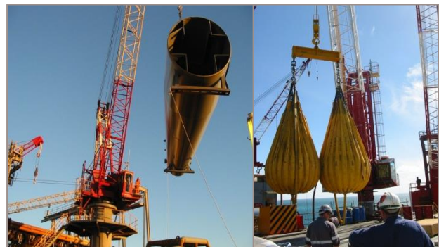
Seatrax 6032 Crane Pedestal Installation and Load testing
