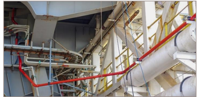
3" Gravel Pack line below drill floor
