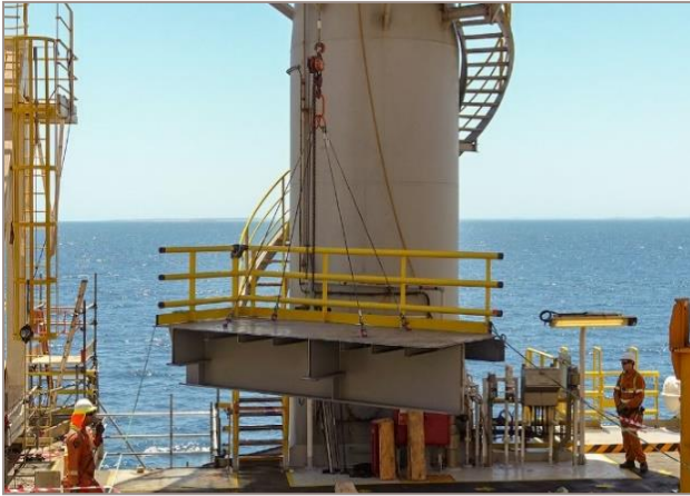
Deck Infill being lifted into place
