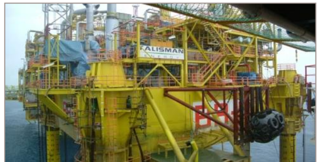
MOAB topside elevated into position
