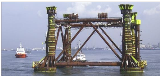
Substructure under tow
