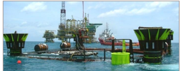
Substructure during ballasting for installation
