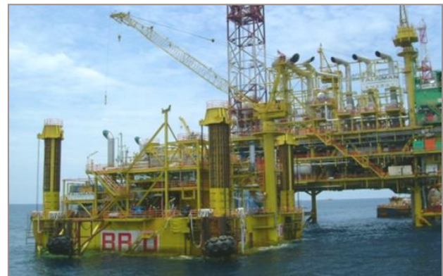
MOAB topside floated over substructure
