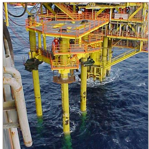
The completed BKA Annex Platform
