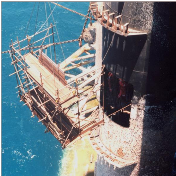
Lifting the prefabricated scaffold into place
