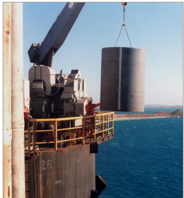
Lifting a section of the chain locker through the deck opening
