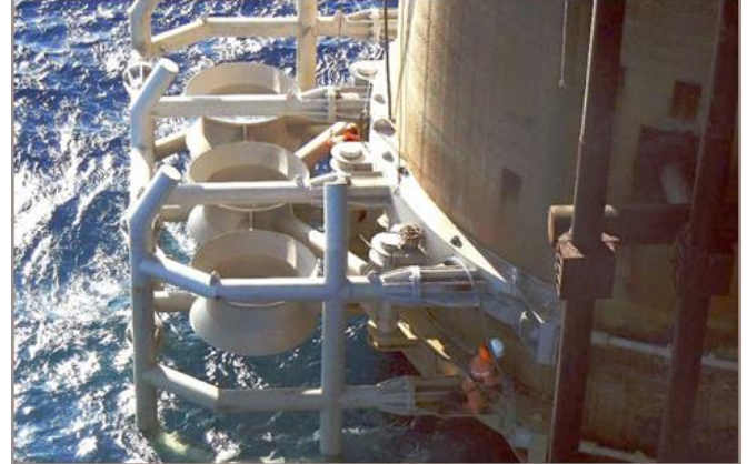
Completed conductor guides and riser protection
