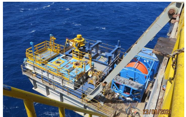
Subsea equipment deck
