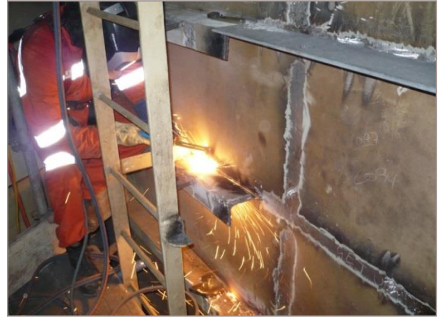
The “Sirius” self-elevating platform located alongside the Double Island platform during installation
