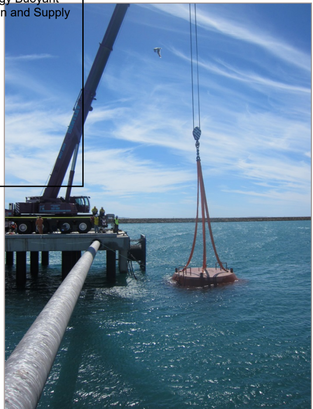
Installing the Buoyant Actuator
