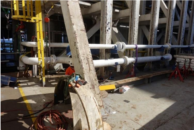
Installation of 6" and 8" relief line spools in the well test area
