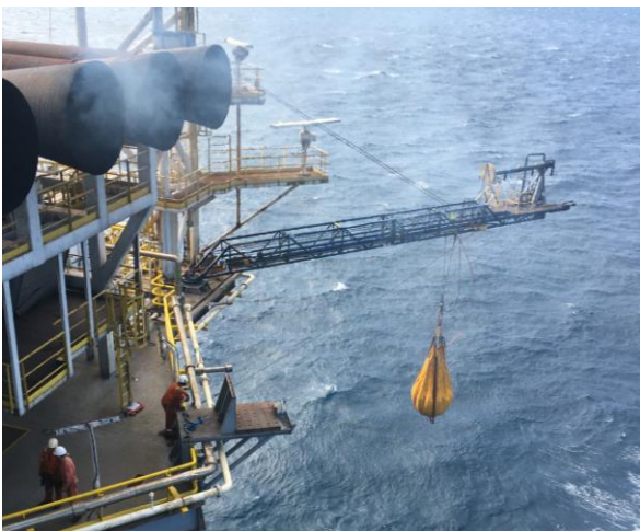
60ft flareboom installation and load testing
