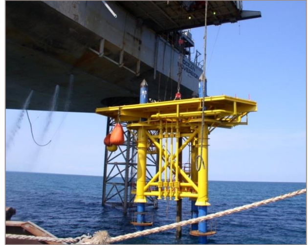
STS Stabbed over 30" Conductors. Production Module not yet installed
