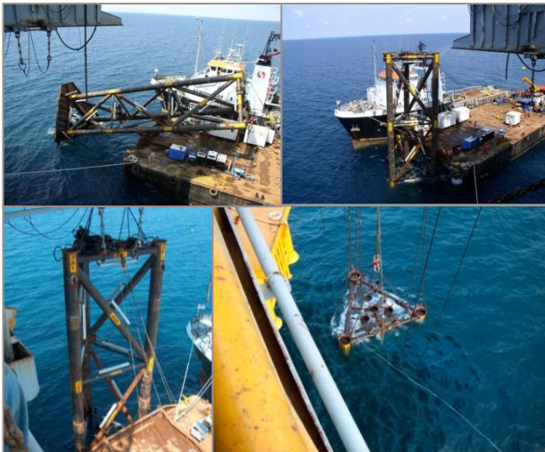
TTS Up-Ending on Barge and Installation onto Seabed
