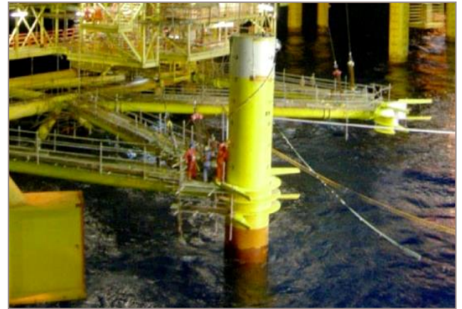
First monopod located into lateral braces
