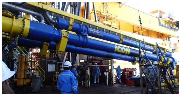
The ARTP E-Series during rig up in the derrick
