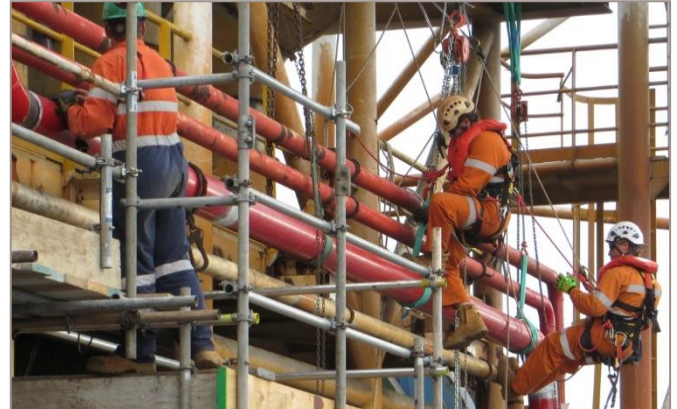
Use of task appropriate access solutions.
