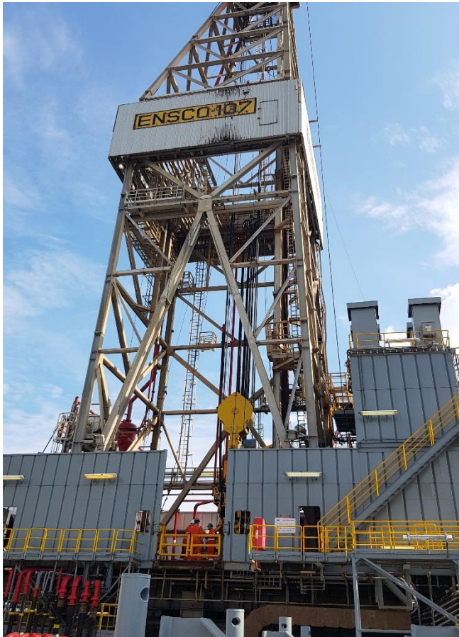
The EnSCO 107 required a significant amount of engineering work to suit the client's proposed range of activities.
