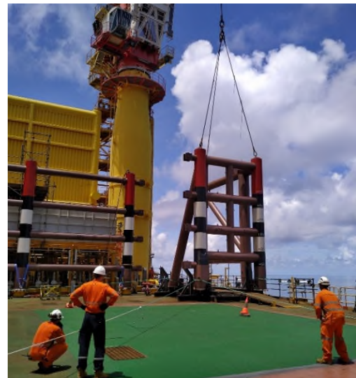
South Panel 1 Land out onto Skidding System.
