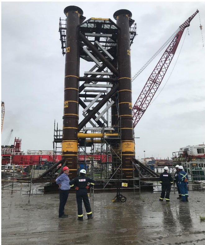
CSP Template at Quay Side, pre-loadout
