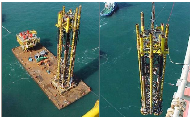
Transportation arrangement and Jacket Lift-off
