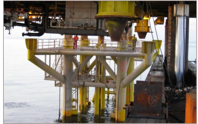
View of Floatover Operation
