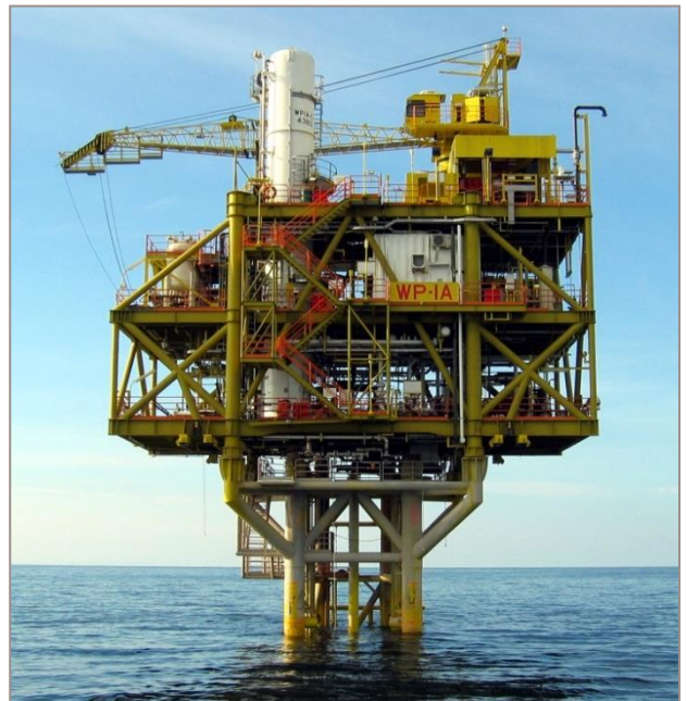
The completed WP-IA platform
