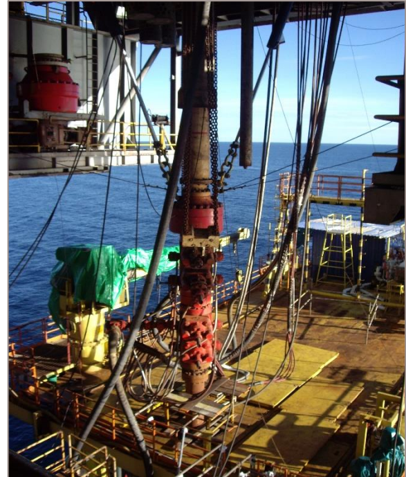
Top Tensioning Drill Floor Installation
