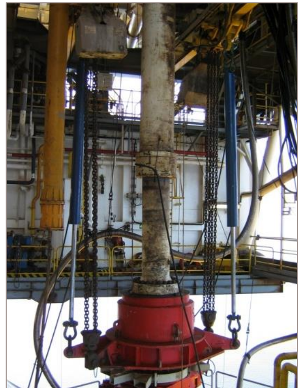
Top Tensioning BOP Crane Installation
