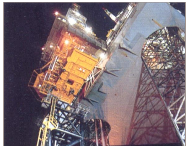
Preparing to lift the upper substructure with sling through the topsides
