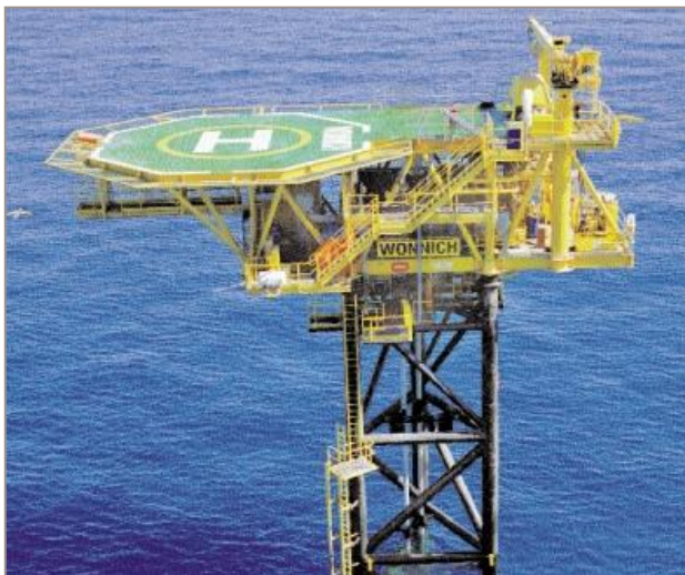
The completed Wonnich platform
