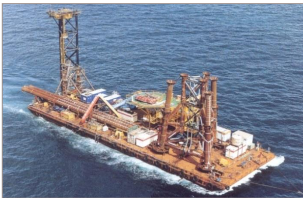
The complete structure was loaded out and transported to site on a single barge
