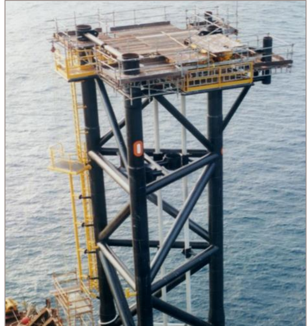
The upper substructure was transported vertically attached to the stern of the barge
