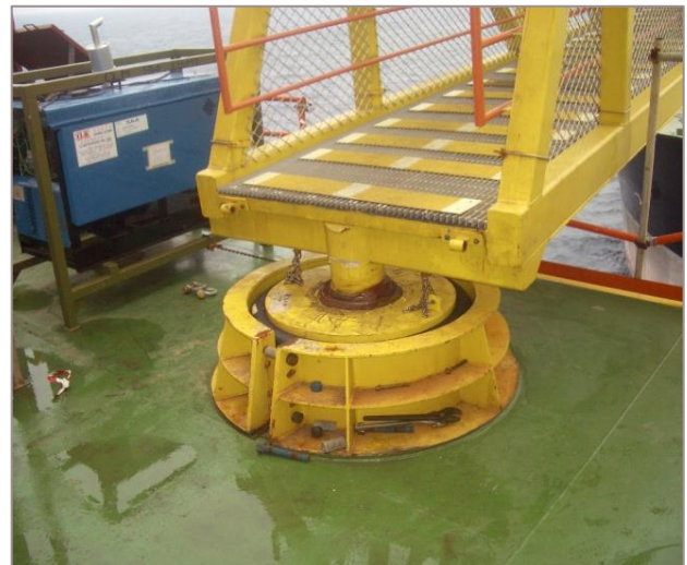
Pivot Bucket support of dynamic bridge (step removed)
