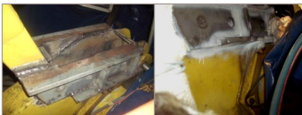
Partial repairs by other contractors were assessed and integrated
