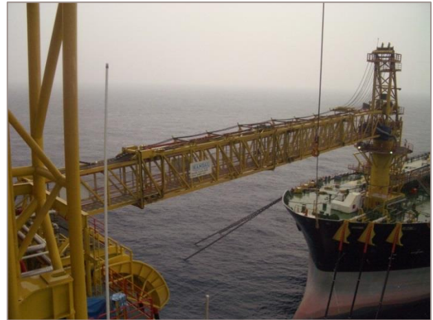
Angsi FPSO to South Angsi A Dynamic Bridge
