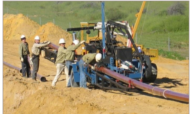
Construction of the GRE Eremia production line to Hovea
