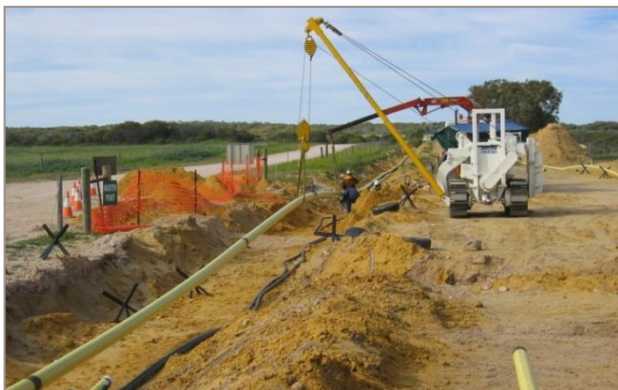
Construction of the XAGGS flowline, which connects various remote fields to the Xyris gas plant facility
