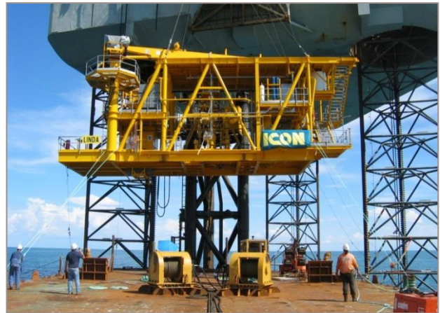
Installation of Linda Topsides
