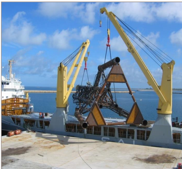
Lifting of Linda Jacket onto HLV for Transport to Dampier
