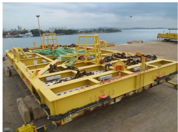
Completed Gravity Base
