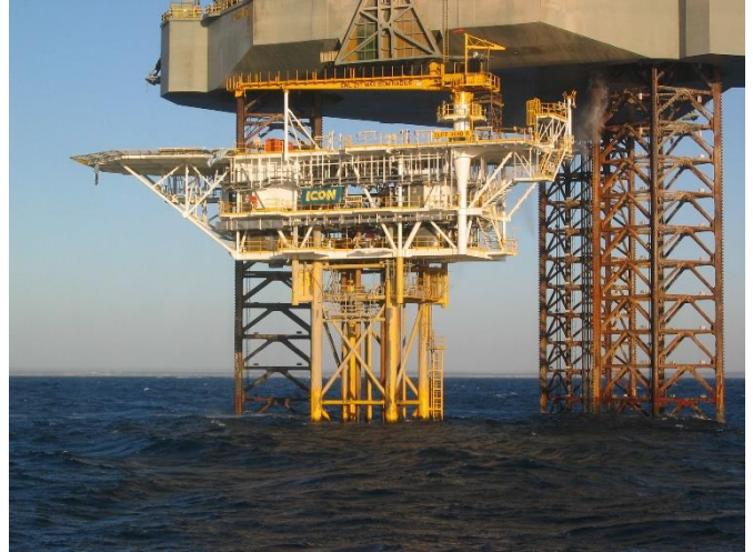
The Cliff Head A platform being originally installed by ICON in 2006.
