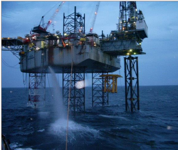
STS hung off aft transom with TTS ready for lowering to seabed
