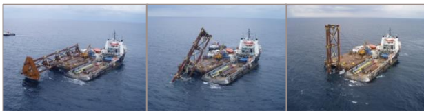
TTS Up-Ending on Barge
