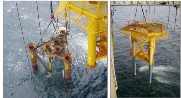
TTS lowering to seabed
