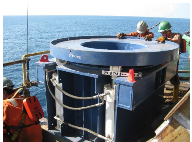
Rig Installed ICON CTUs
