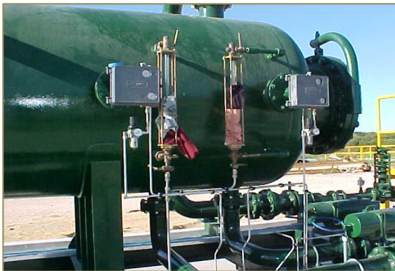
The initial 8,000 bbl/day 3 Phase Separator.
