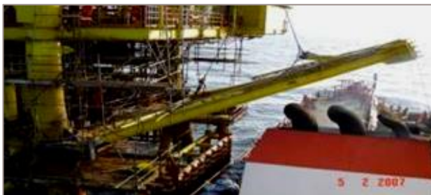
Brace being installed on existing BKC Platform
