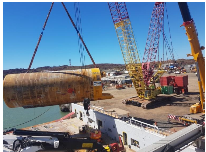
Back loading of the CAN at King Bay
