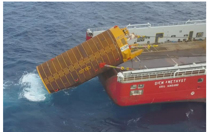
Over boarding CAN from vessel
