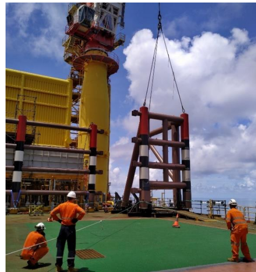
South Panel 1 Land out onto Skidding System.
