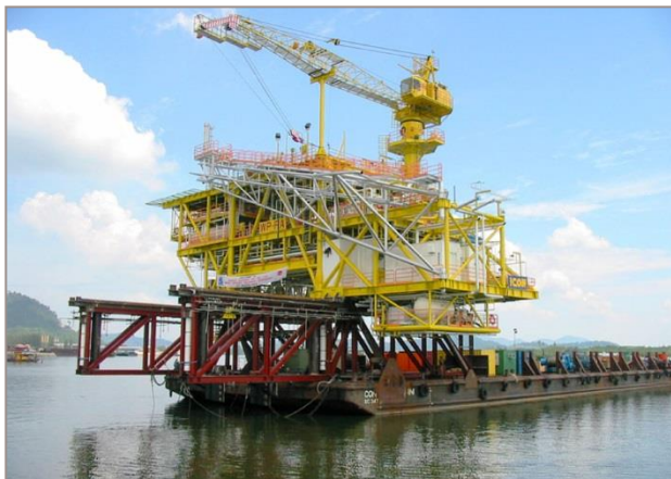
WP-PA Topsides after Loadout – Inboard Transport Position
