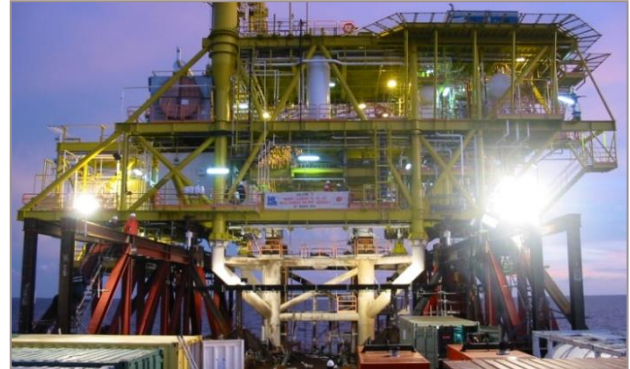
View of Floatover Operation from Barge Deck (Jacket is White)
