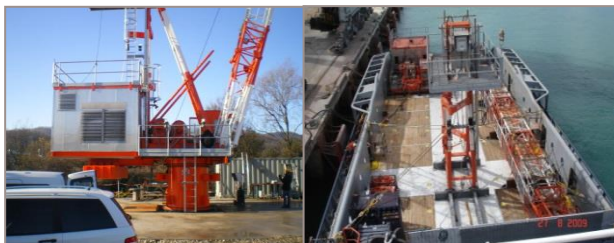
Trial assembly shore side / Sea fastening for voyage
