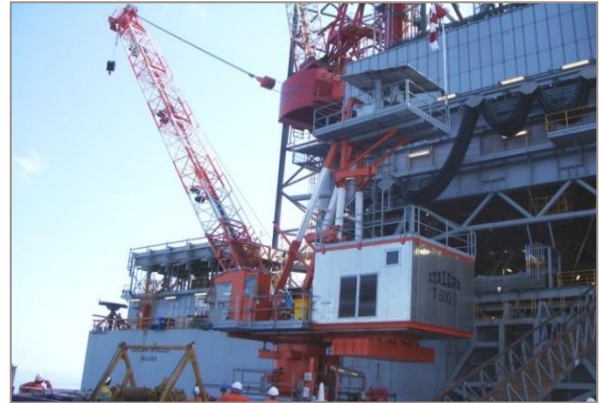
Blacktip crane installed and tested
