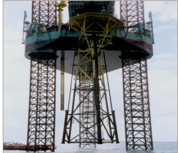
Installation of the Buffalo WHP by ICON using a Jackup Rig
