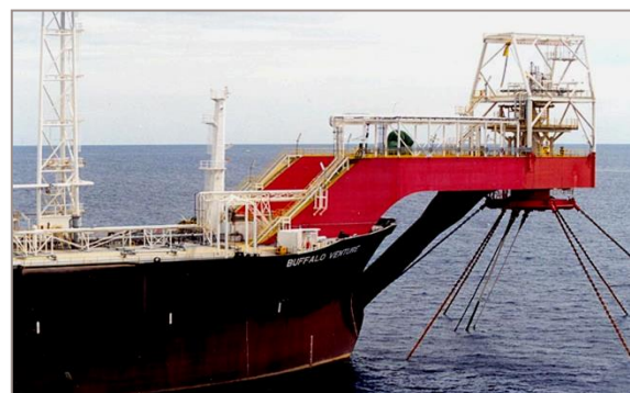
Buffalo Venture FPSO 6 Point Mooring, Riser and Control Umbilical
