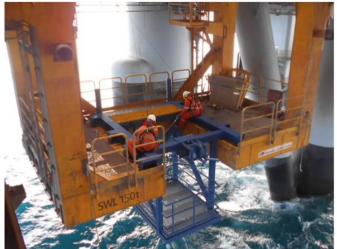
Blue ‘shark cage’ installation.
