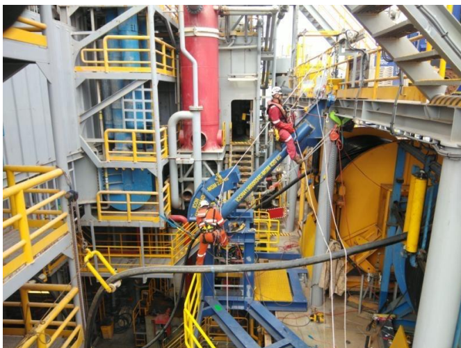
RATs installing the Sheave Support Structure over the moonpool: Elevation View.
