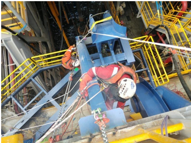
RATs installing the Sheave Support Structure over the moonpool
