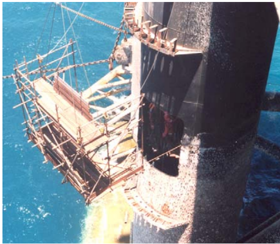
Lifting the prefabricated scaffold into place.
