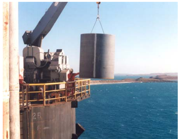
Lifting a section of the chain locker through the deck opening
